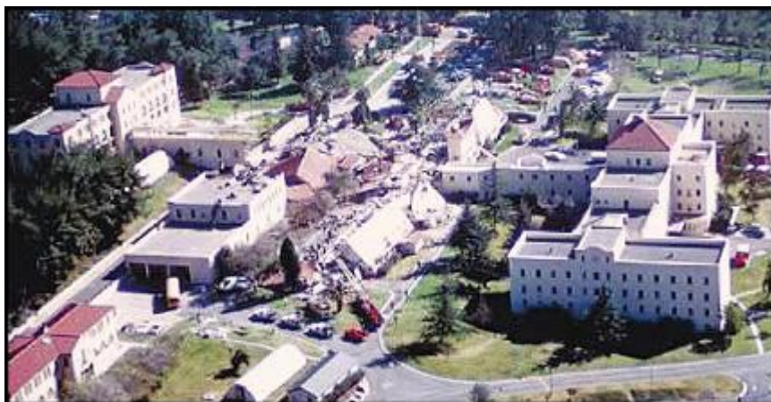
San Fernando Medical Center collapse, 1971
